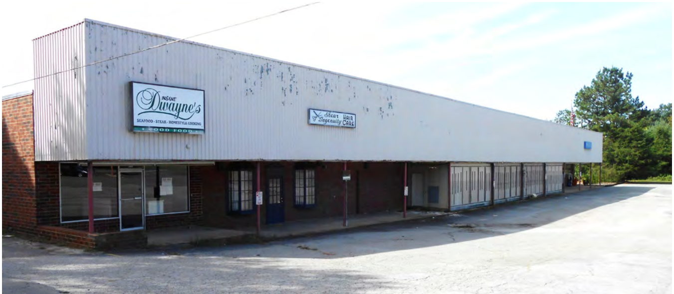
▼ IMAGE 3.14 UNDERUTILIZED STRUCTURE ON MAIN STREET
