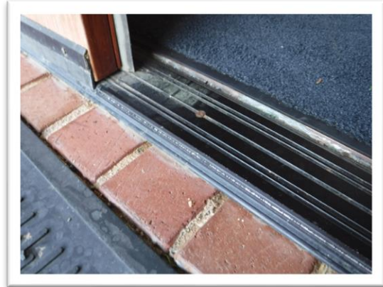
Figure 1: Entrance 1 (Approx. 0.48", 67% Slope)
