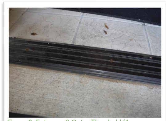
Figure 3: Entrance 3 Outer Threshold (Approx. 0.48", 85.3% Slope)
