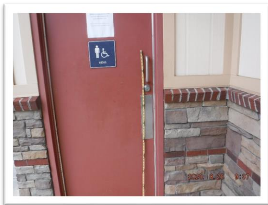
Figure 15: Park Male Bathroom Hardware Height
