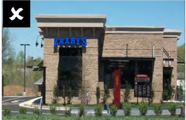
Drive-through ordering station on primary facade
