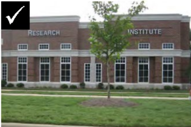
Continuous parapet with height changes
