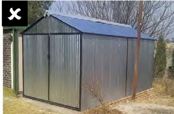
Materials do not match principal structure
