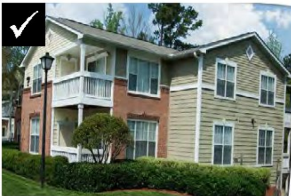
Adequate windows with regular rhythm and alignment
