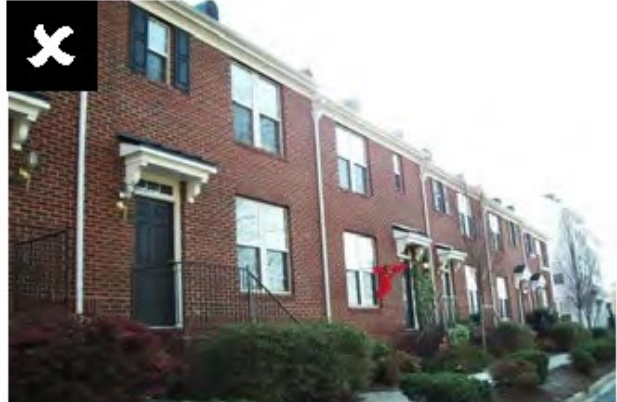
No facade articulation
