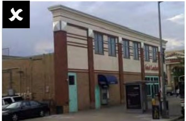
Non-continuous parapet without height changes
