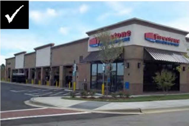
Service bays on secondary building wall
