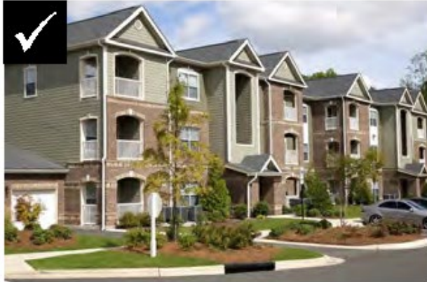
Facade articulation with recesses and projections
